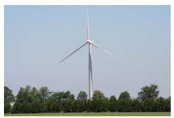
Wind turbines produce noise from two distinct sources; the sound of rotor blades as they rotate (aerodynamic effect) in the wind and the motor noise from within the turbine unit itself (mechanical operations). The sound wind turbines emit is described as audible or as infrasound, that which is
